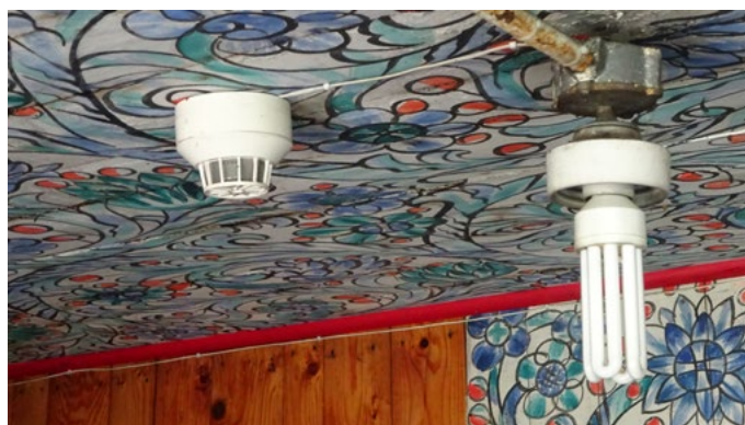
2. Smoke detectors (above) and an unsecured lamp on the wooden ceiling of a larch church (below) © Krzysztof T. Kociołek
