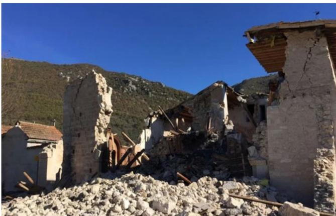
8. *San Salvatore Church, after Central Italy earthquake, 26 Oct. 2016. The aftershock on October 30, 2016, caused further collapse of the remaining left part of the facade and the wall between the two naves* © Silvio Sorcini - Wikipedia
