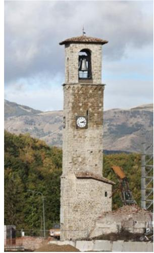
15. Amatrice, Civic Tower, before and after the 2016 Central Italy earthquake; reconstruction and restoration works (2022-2023). The stone blocks recovered from the rubble of surrounding buildings (Type B debris) were reused for wall reintegration and the masonry cladding of the new bell tower © Maria Agostiano © Corpo Nazionale dei Vigili del Fuoco
