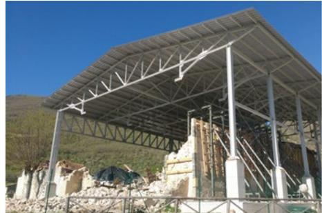
10. Securing lateral wall ruins with a temporary steel cover and bracing, April 2017 Wikimedia Commons
